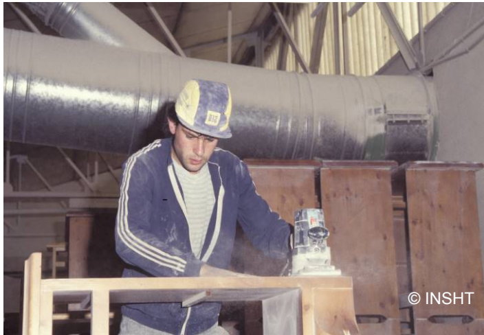
Young worker exposed to wood dust
